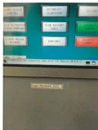
“Connection open error” on RAS display screen. Manufacturer is out of business, we are researching options for a fix. All pumps remain operational we just lost flow data for internal plant recirculation.
