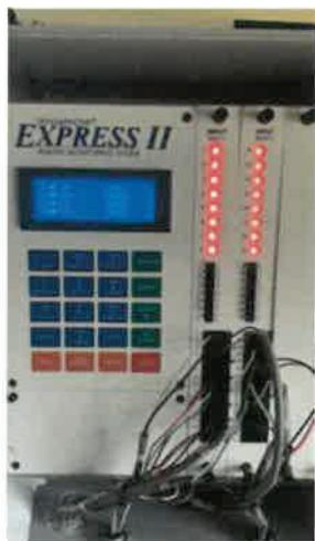
Alarm System malfunction turned out to be old backup battery connection. Battery has since been changed; alarms are all functional.
