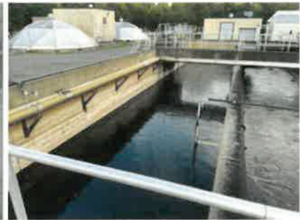
Biosolids Storage Tank
